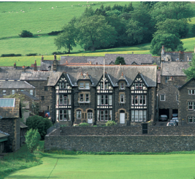
2001 The building now called Lupton House was built originally by a local builder as three terraced houses and called Jackson's Buildings. Lupton received its fixed name in 1908 and is named after Roger Lupton, the founder of Sedbergh School. It was closed as a boys' boarding house in 1995 and became the Lupton Centre until 2001. It was then reopened as a girls' boarding house.
